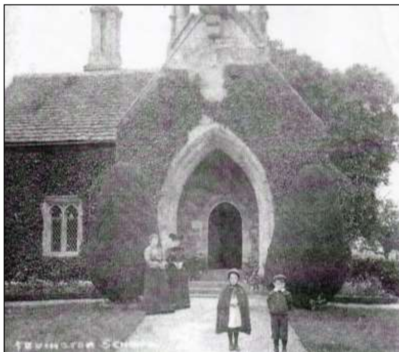
4. Sevington School Exterior
